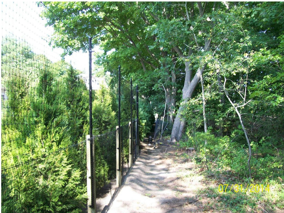
Compliant pool enclosure fencing on 4 X4's. Black metal posts with plastic mesh deer fencing above.
